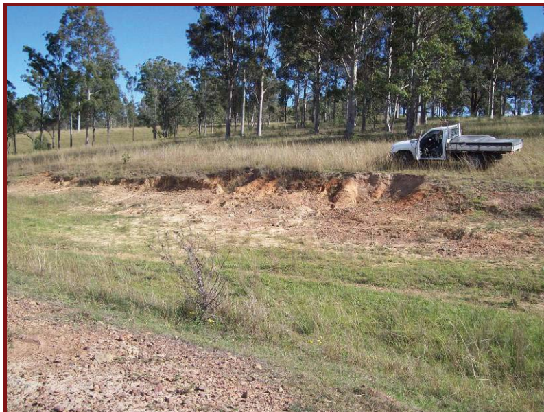
Photo 14 – Localised minor erosion in the central portion of the site
